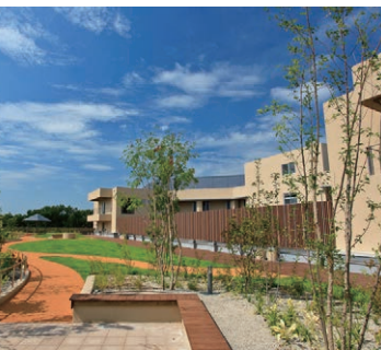
Hospital rooftop garden
